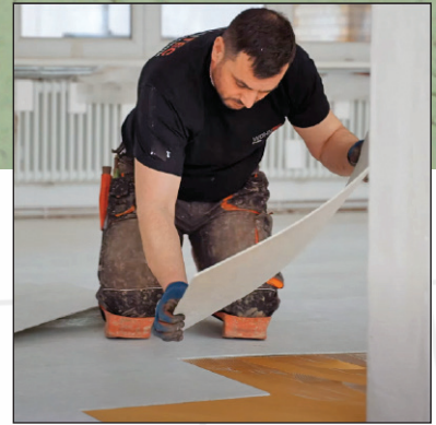
Stagger the panels to eliminate long seams.
