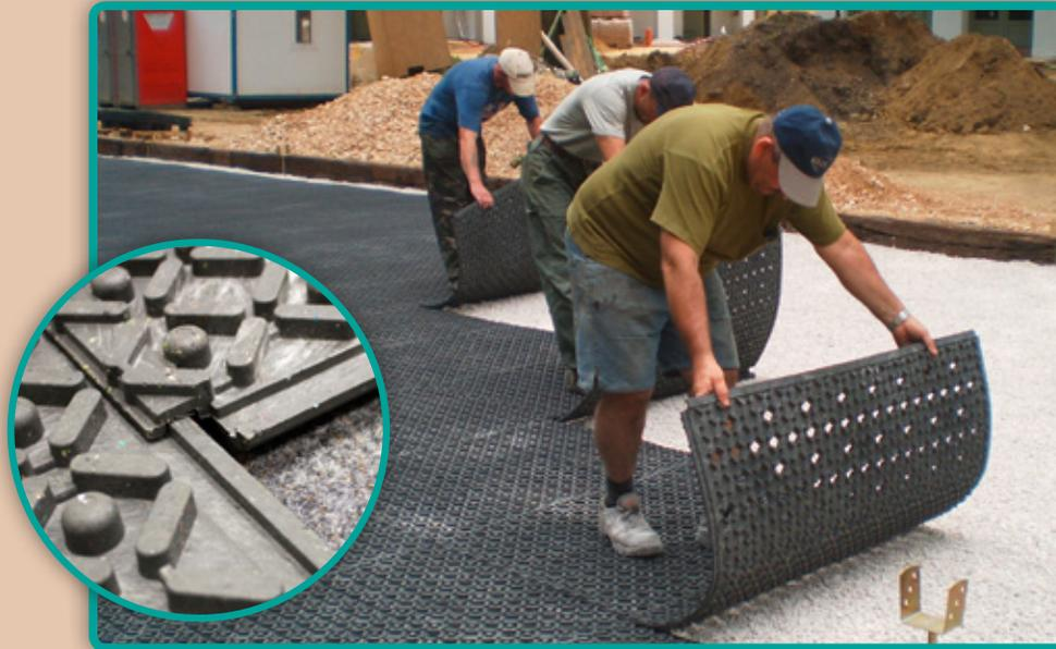
should keep drainage open and prevent the fine top footing sand to be washed thru the mats out of the arena.
